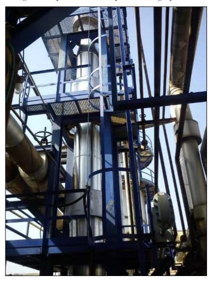
Figure 2: Wiped Thin Film Evaporator during Operation
